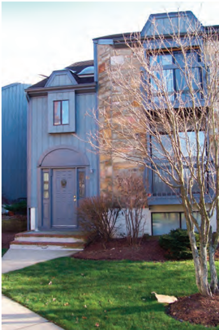
This residence was donated to Community Hope to provide housing-plus-services for three adults in recovery.
